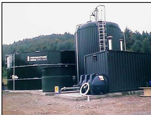
Figure 2. Biogas Plant (Anaerobic digester and waste storage tank).
