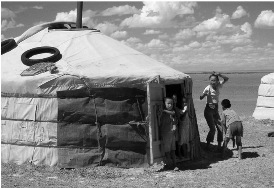
The felt covering for the roof and the lattice walls can be clearly seen; the front door is on the right hand side.
