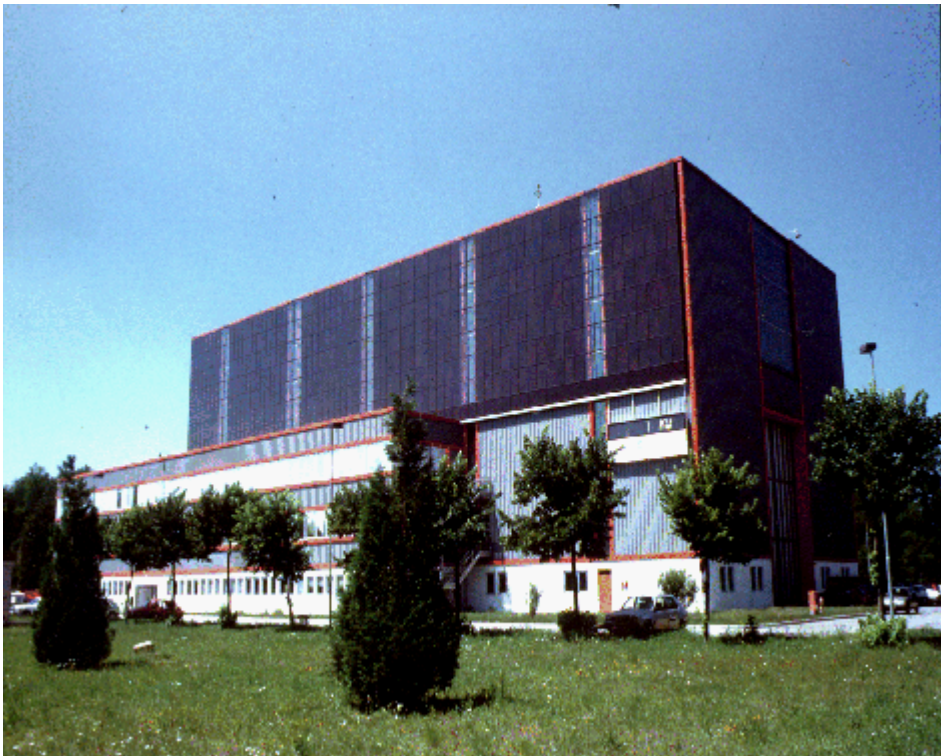
Figure 6: Focus of scaling example: the ELSA building, Ispra
