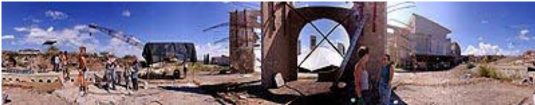
Arcosanti: East Crescent under construction, 1999
