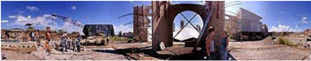
Arcosanti: East Crescent under construction, 1999
