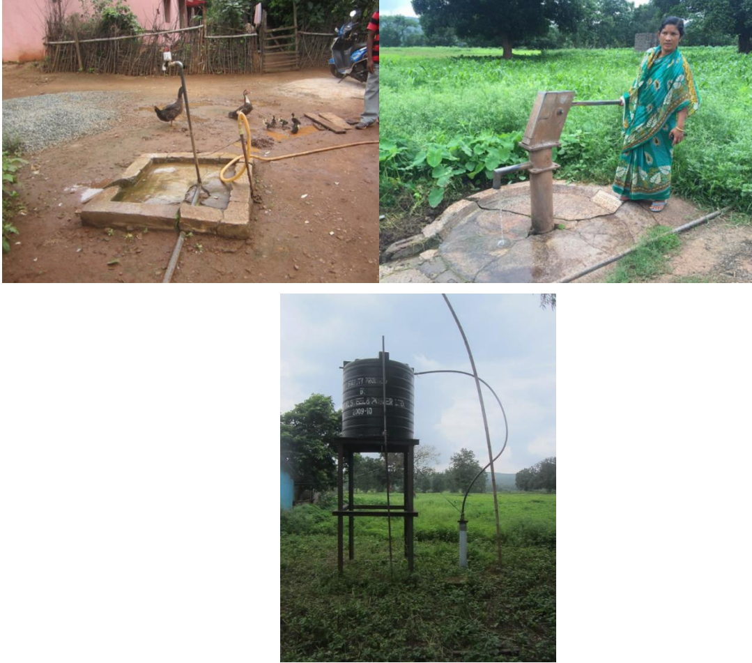
Figure 10: Clockwise - Public stand post, public hand pump and public bore well in Lahanda and Kaliabeda villages.
