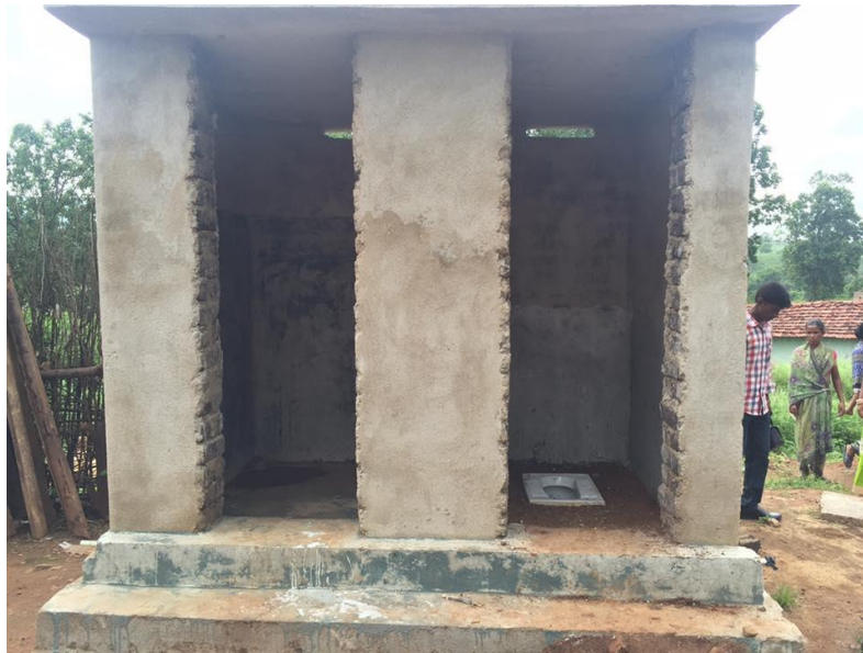
Figure 12: Toilet and Bathroom Superstructure Initiated by Gram Vikas
