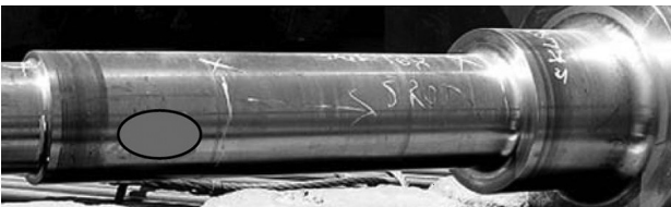
Figure 11: Detail of extent and location of the defect on the generator rotor shaft – forging No. 447 660 Slika 11: Velikost in mesto napake na gredi rotorja generatorja – odkovek št. 447 660
