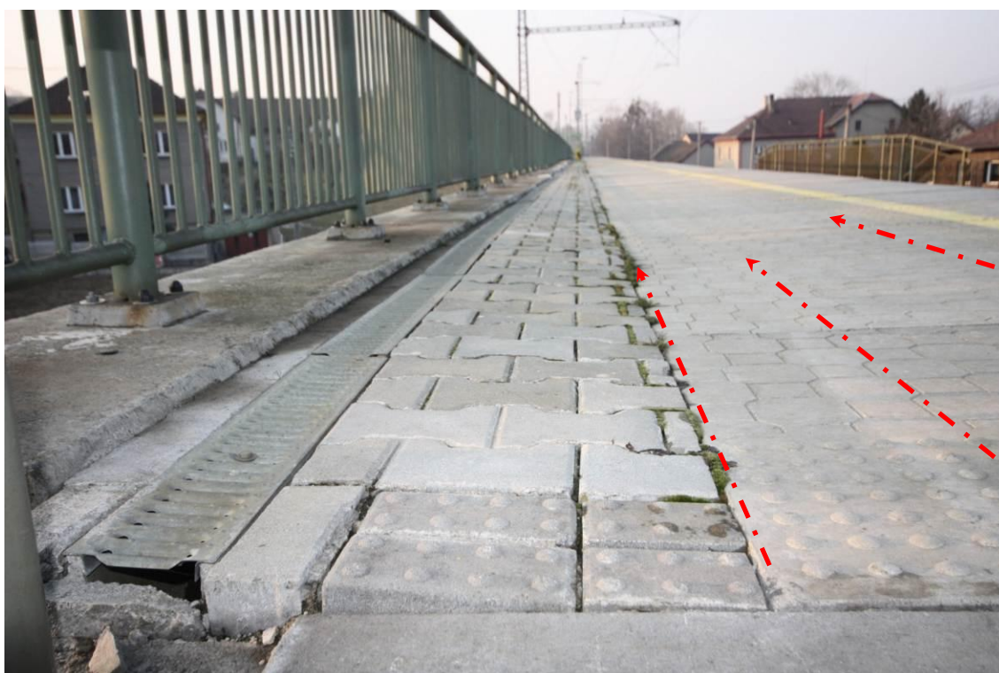
Fig. 9 Schematic representation of the directions of 3 parallel radar profiles, spaced 80 cm (used antennas with a frequency of 250 MHz and 500 MHz). Photo A. Poláček.
