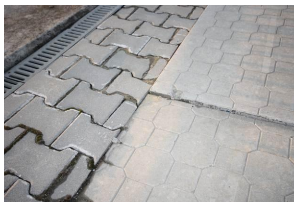
Fig. 7 Detail of the platform surface deformation at the interface between interlocking pavers and concrete panels. Photo A. Poláček.
