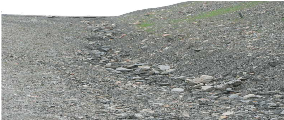
Fig. 3 Maintenance of inclined roads and benches
