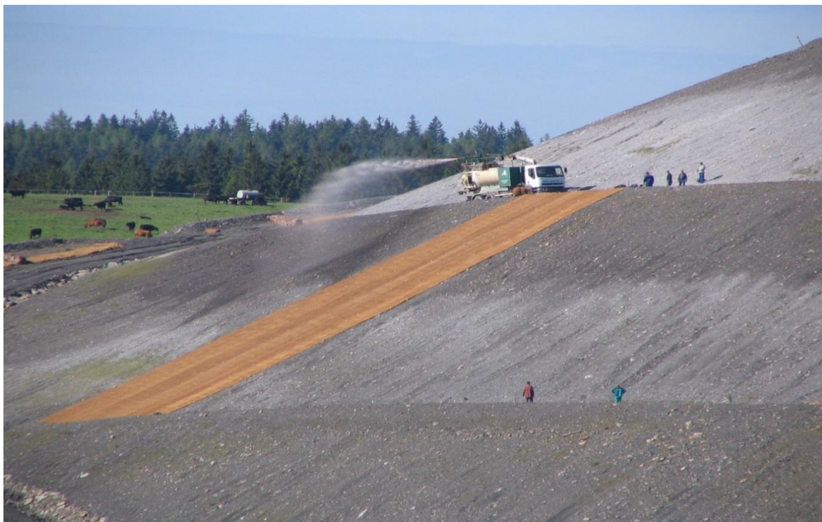
Fig. 4 An example of hydro seeding and coconut mats
