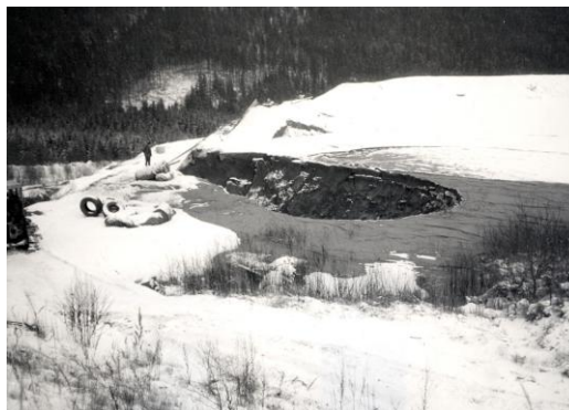
Pic. 3 Dam failure in Zlaté Hory
