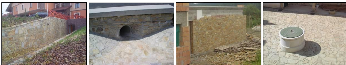
Figs. 8, 9, 10, 11: Examples of course stone products used for engineering-type constructions
