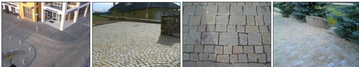
Figs. 3, 4, 5, 6: Samples of road construction program
