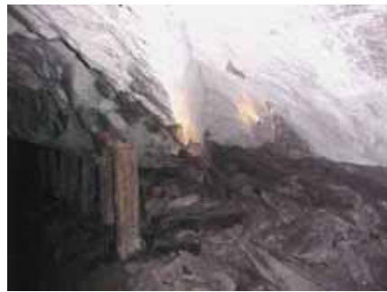
Fig. 15 A shake-up of hangingwall after seismic event caused detachment of rock from prominent joint (still contained within the siding)
