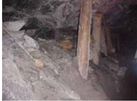
Fig. 13 In most instances sidings blasted next to the ASG (advanced scraper gully) contain the fractured rock
