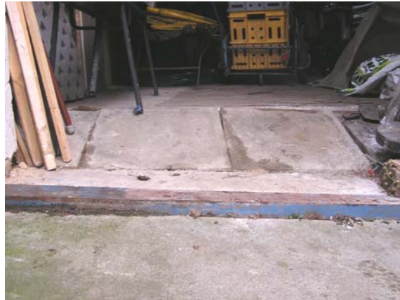
Fig. 9: Bent fence in the top part of the slope deformation (left) Figure 10 Terrain deformation with the manifestation of floor bulging in the workshop up to 15 cm (right)
