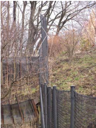
Fig. 9: Bent fence in the top part of the slope deformation (left) Figure 10 Terrain deformation with the manifestation of floor bulging in the workshop up to 15 cm (right)
