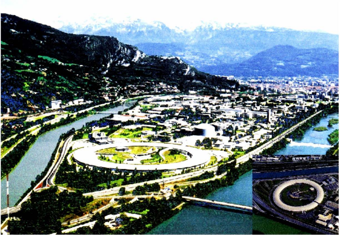
Figure 3.5. The ESRF, Grenoble, France. Steep overhead view given in inset. The circular storage ring of the electrons can clearly be seen. The strip extending into the storage ring is the linear accelerator (linac), used to initially boost the electrons up to speed before circulation.
