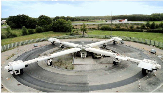
Fig. 1 Accelerated pavement testing facility of IFSTTAR.
