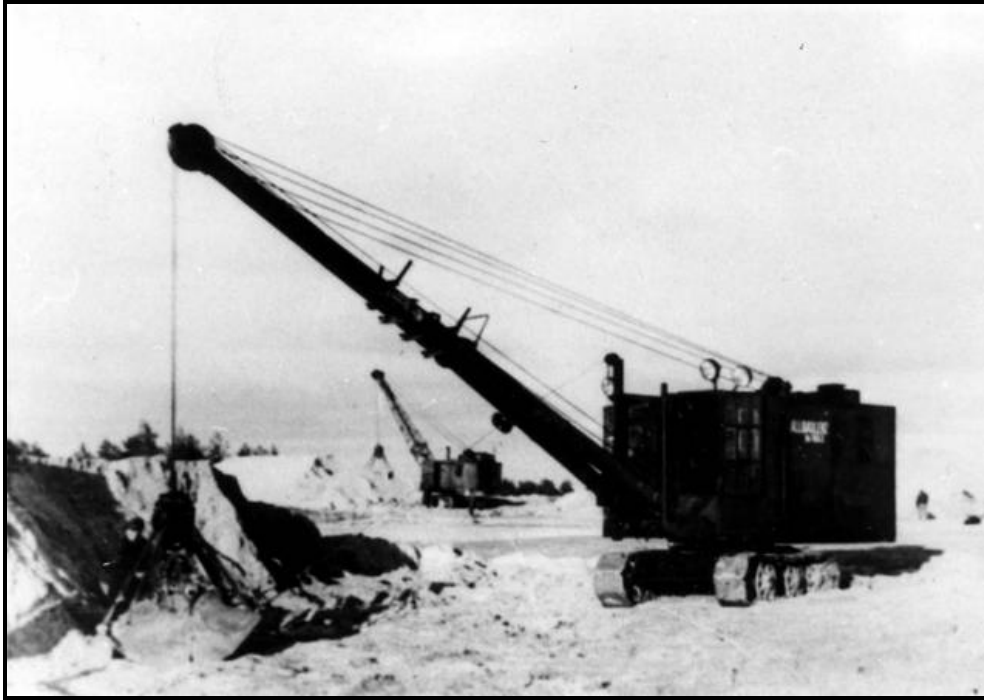
Plate 4.27. Excavators or 'kopachke' used to dig some of the graves at Treblinka II (after YV 1448c)
