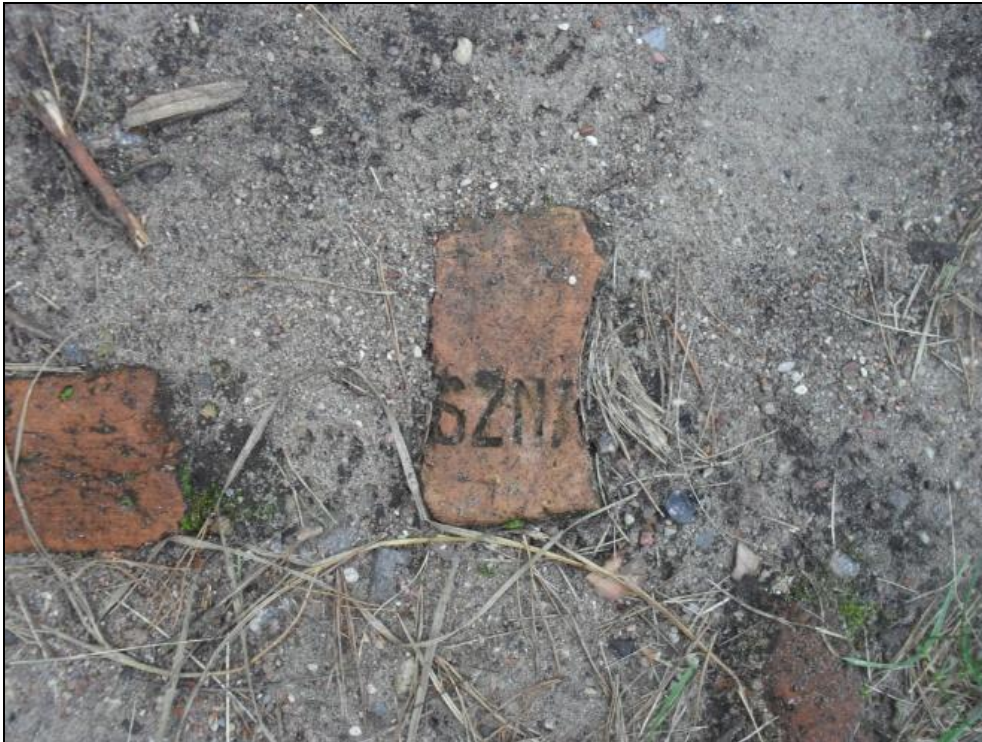
Plate 4.24. Bricks noted in the region believed to have contained the Ukrainian guardhouse (author's own photograph)
