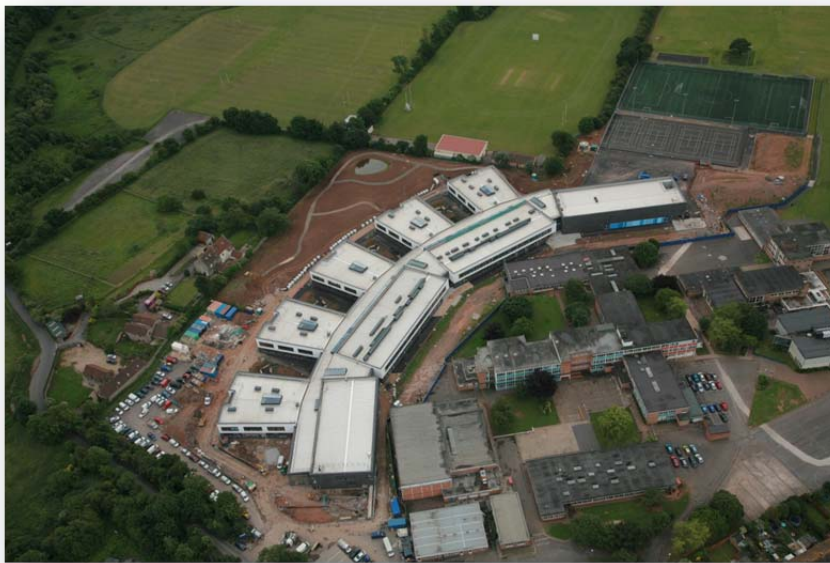
Image 6.1: BEC: Aerial view showing the new school (centre) and the old school (right) Courtesy of Atkins (2009)
