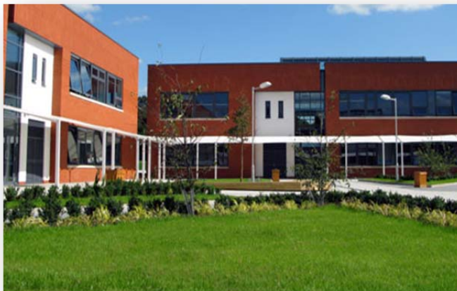
Image 9.3: BWS: Facade Courtesy of NCC (2010)
