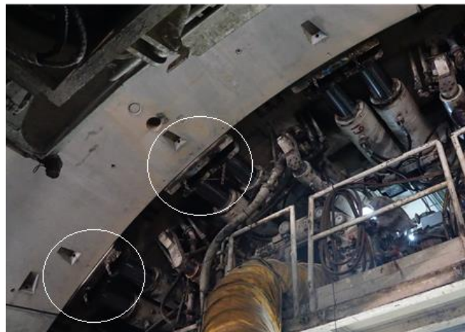
Figure 4.3 Radial eccentricity of hydraulic jacks in the L9 metro line in Barcelona.
