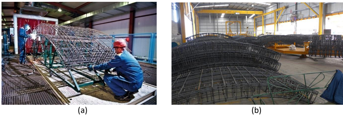
Figure 5.5 Tunnel segment reinforcement construction (a). Reinforcement storage area (b) ( http://www.tunnel-online.info/en/artikel/tunnel_2011-01_Steel-fibre-reinforced_segmental_linings_State-of-the-art_and_completed_1076896.html ) ( https://www.tunneltalk.com/Mexico-City-Emisor-Oriente-30May13-Mega-drainage-project-site-visit-report.php )
