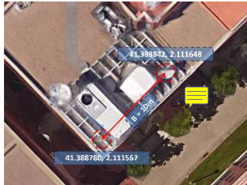
Figure 5 (Color online) Zenith view of the receiver locations at the UPC Campus Nord D3 building.
