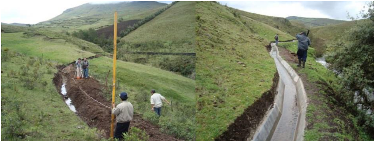
Figure 2. Construction of the micro-hydro power plant of El Regalado, Peru [31]
