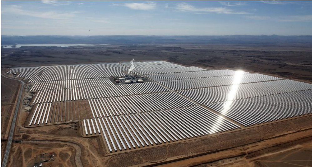
Figura 5.12 Central termosolar Noor I-Ouarzazate. [45]
