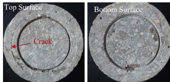
Fig.7 Cracking of a specimen with height of 80 mm suggesting the deviation of the main crack
