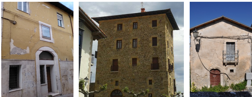
Figure 4: Examples of URM walls with irregular configurations.
