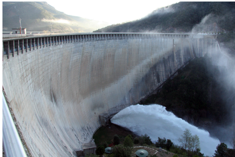
FIGURE 5.1: View of La Baells dam.
