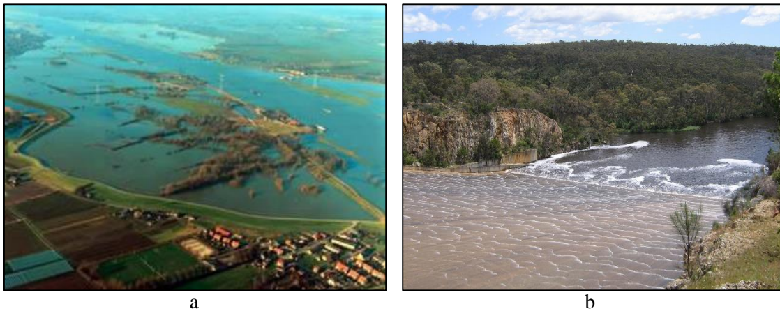
Figure 4.1.5. a) Afferdense waard during a flood. Mild slope, normal flow is subcritical. (Blom, 2015); b) Spillway Para dam US. Steep slope, normal flow is supercritical. (Blom, 2015)
