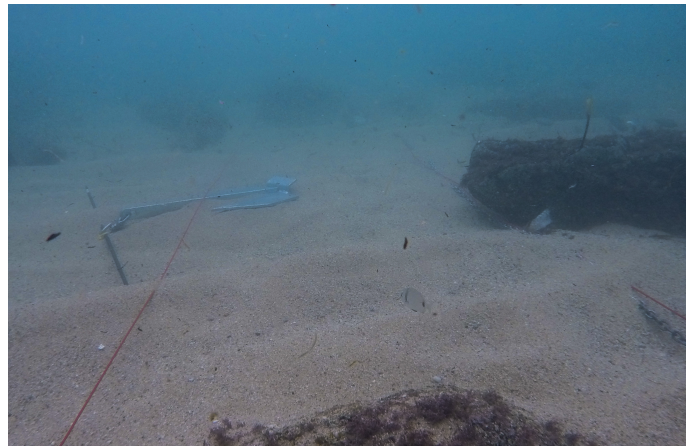
(e) Placement of the submerged optical fiber
