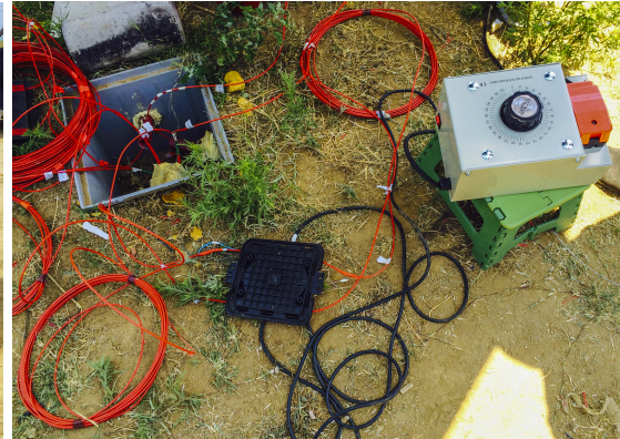
(b) Pit with piezometer and optical fiber (in red)
