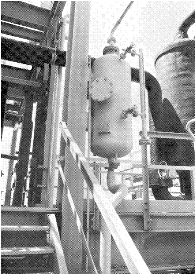
Figure 11. Overhead Seal Differential Pressure Tank.
