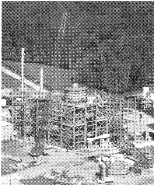
Figure 1. Hersey Plant Site Under Construction.
