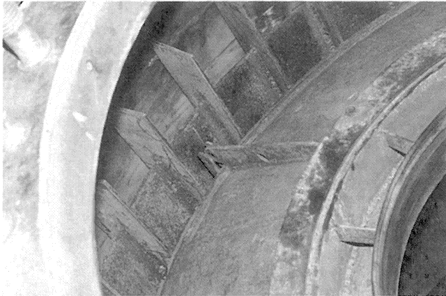
Figure 78. Photograph of Struts with Missing Clevis Pins.
