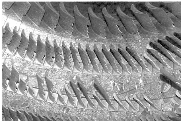
Figure 72. Lower Casing Stator Section Damage.
