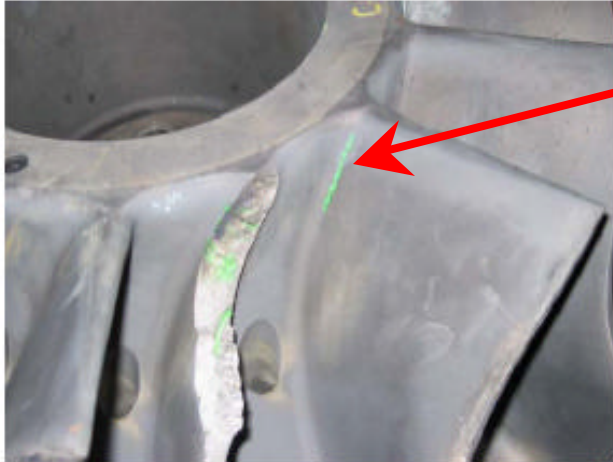
Macro photograph (flash and black light) showing the secondary crack in the radius of the adjacent blade to the primary fracture. IMG_4273.JPG
