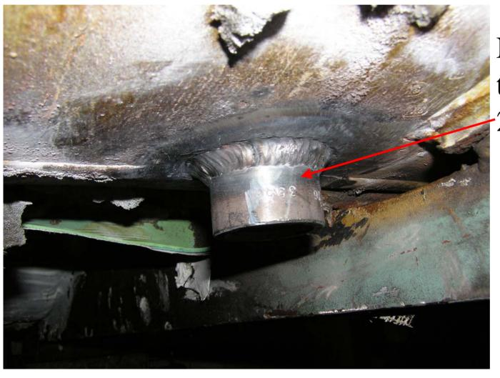
New drain at the rear of the  $2^{nd}$  intercooler
