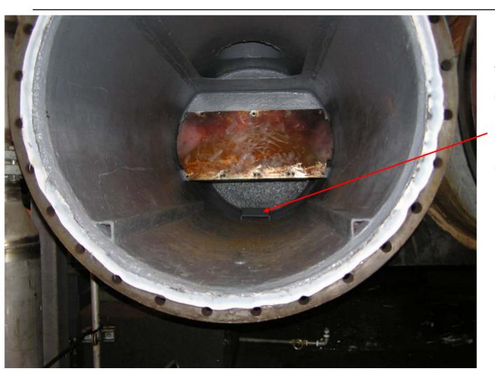
Added baffle/deflector over 2<sup>nd</sup> intercooler drain
