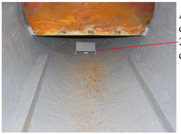
Added baffle/deflector over 2<sup>nd</sup> intercooler drain
