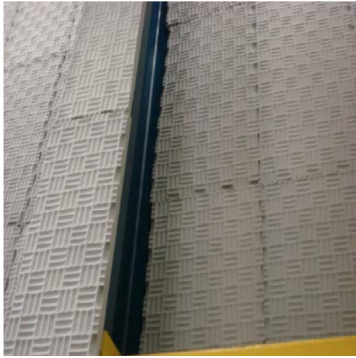
Figure 17. Foam Installation.
