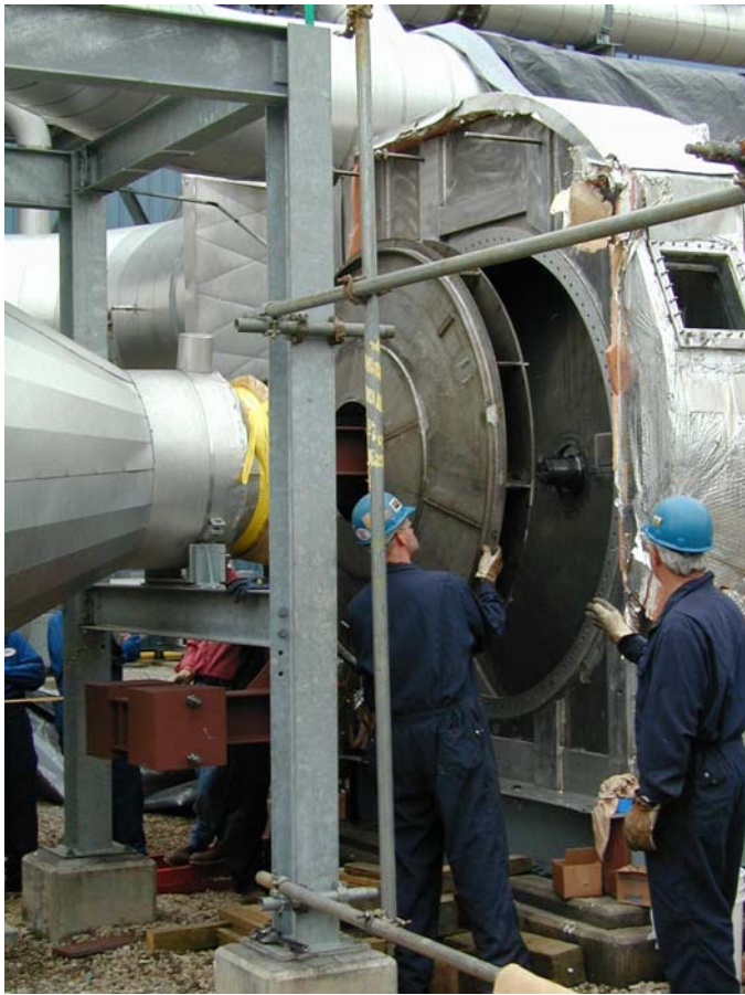
Figure 23. Impeller of an 800 HP fan before measuring the natural frequencies and mode shapes of the back plate.
