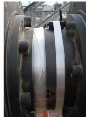
Figure A.2. Strain Gage Telemetry System Installed on Coupling Spool Piece.
