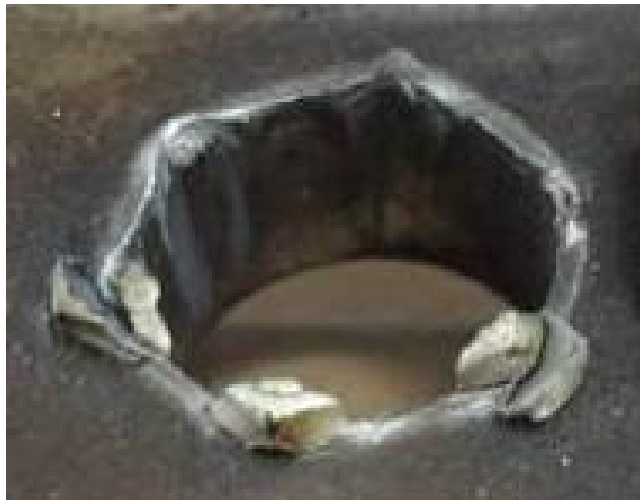
Nut/bolt pulled through flange
