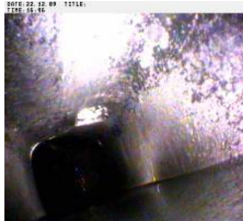
Outlet of long cross over inspected first for obstruction. Nothing found. But what is that we see in the distance?
