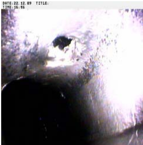
Outlet of long cross over inspected first for obstruction. Nothing found.
