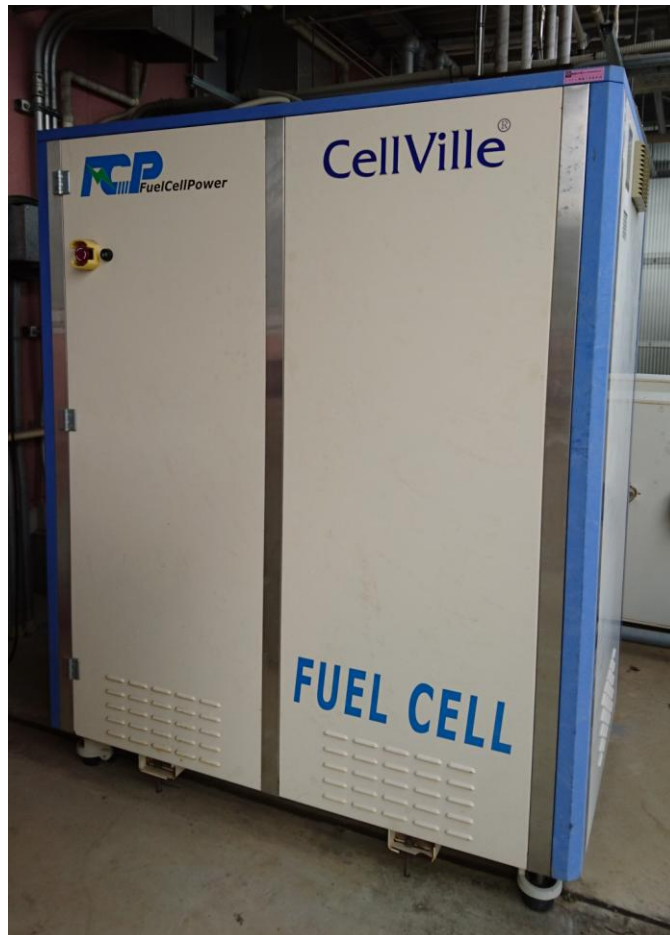
Figure 2.8: The PEMFC 10 kW used in CNES under the study.
