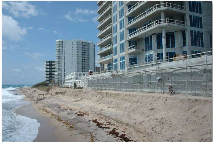
New Construction on Critically-Eroding Beach Singer Island, Florida
