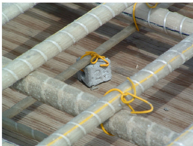
Fig. 1 GFRP bars used for negative and positive reinforcement in bridge decks, Courtesy of Hughes Brothers
