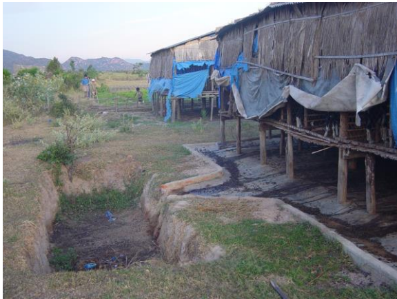
Well designed manure collection system
