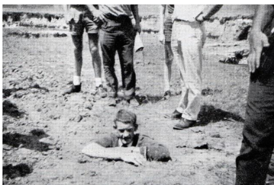
Alan Patterson testing post hole depth
