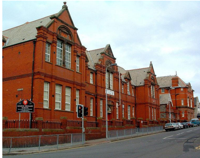
The Holton Road Primary School, Barry Established in 1891
