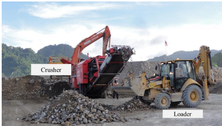
Figure B-2. Sampling crusher discharge
