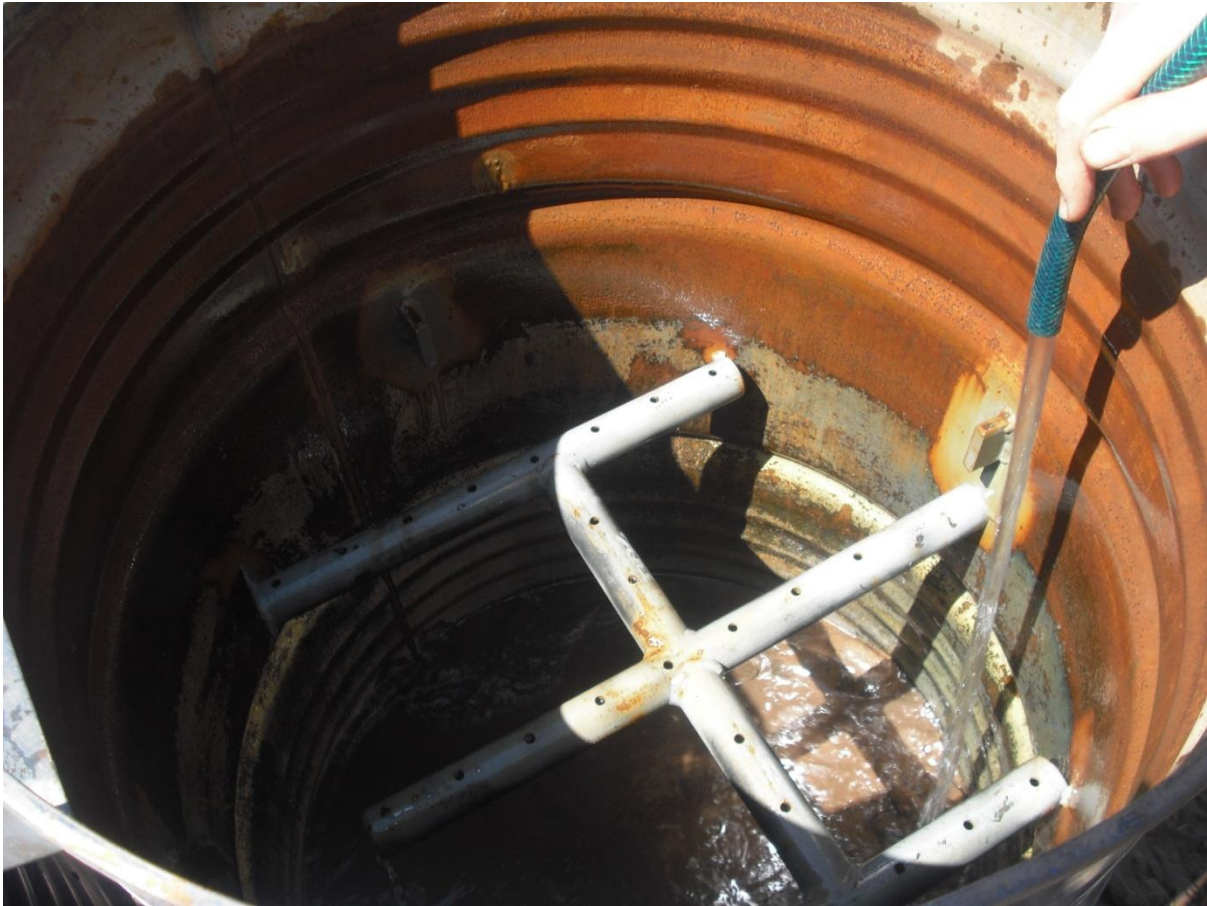
Figure 4.2 The branched assembly inside the main tank at the top of the cascade. Photo courtesy of Gemma Irving.
