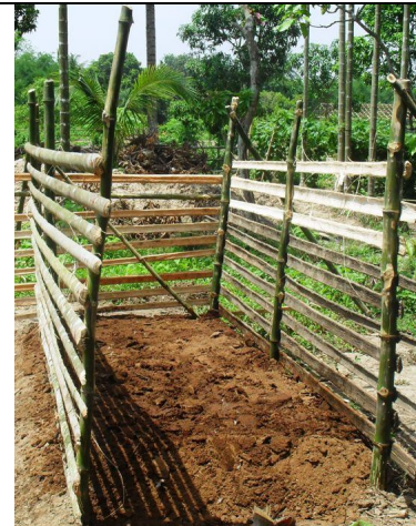
Pic. 1 : Bamboo structure to support the Novcom poultry compost Heap
