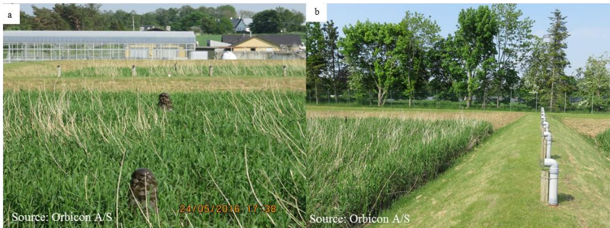
Figure 3.. a) Active loading pipes in an STRB system. The pipes protrude vertically from the sludge residue and ensure the even distribution of sludge over the surface. b) The reject water system underneath the beds is open to the atmosphere (pipes protruding from the ground), thus allowing oxygen to enter the filter layer and the lower parts of the sludge residue.
