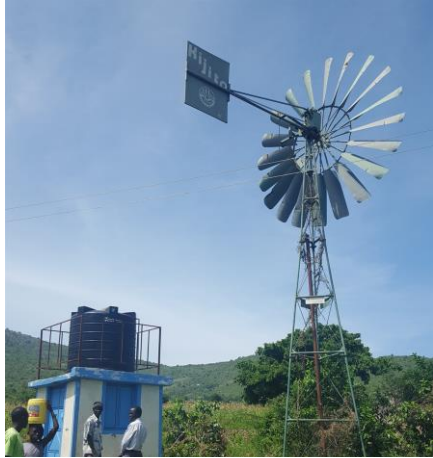
Photo 4: Mechanical wind pumps. Most of the systems have been replaced by solar systems
