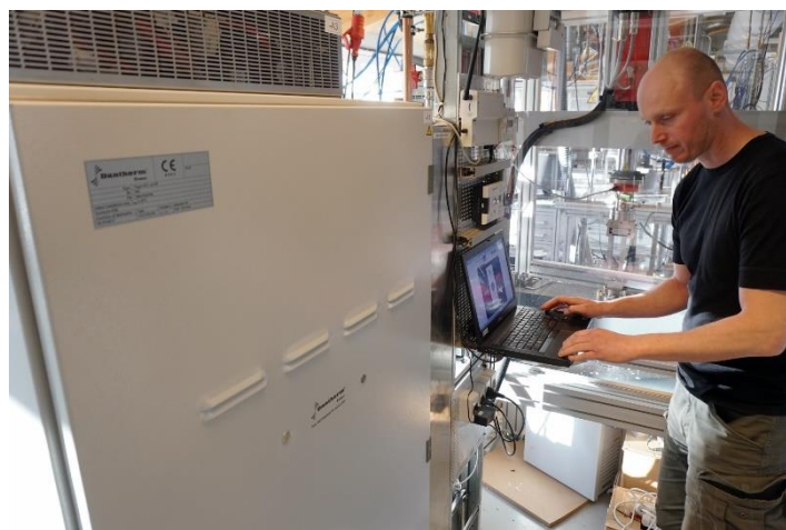
Figure 11. \mu CHP unit at DTU Energy through the EU ene.field project
