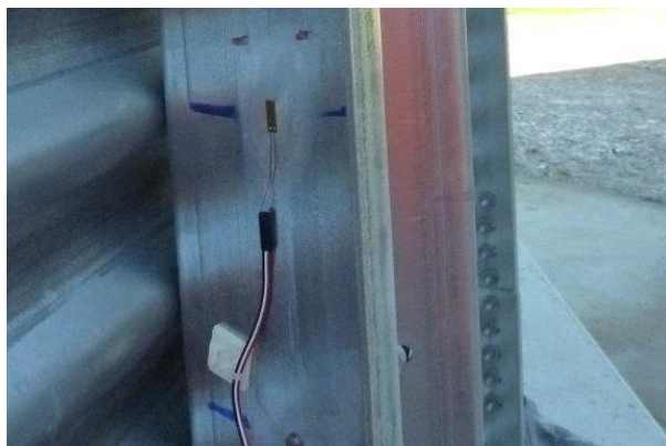
Figure 11.9 – Typology of 8 mm long strain gauges mounted on the silo wall and vertical stiffeners
