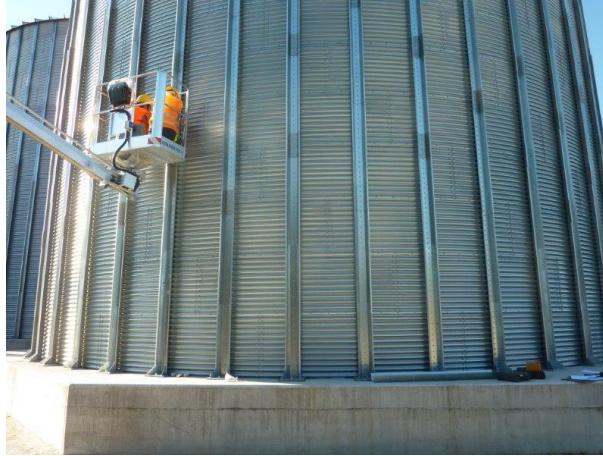
Figure 11.16 - Measurements on the measuring bases on the elevator
