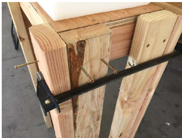
Figure 18: Clamping for Stand Construction
